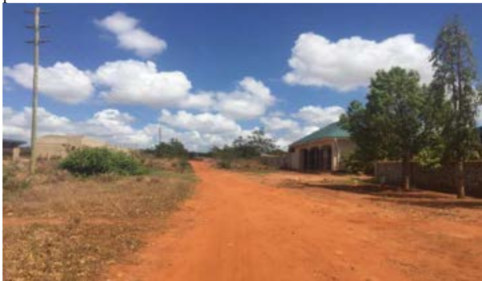
Picture 2-3: Condition of Existing Muhimbili Road
