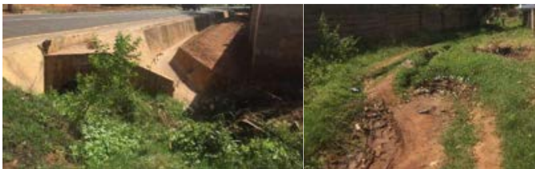
Picture 2-10: Existing Drainage System at Baracuda alone Modeco Road
