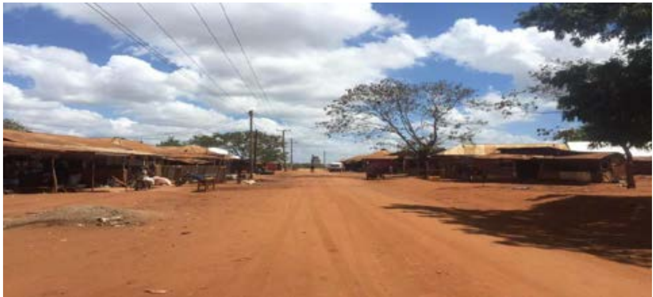
Picture 2-7: Condition of Existing Tubuyu II Road
