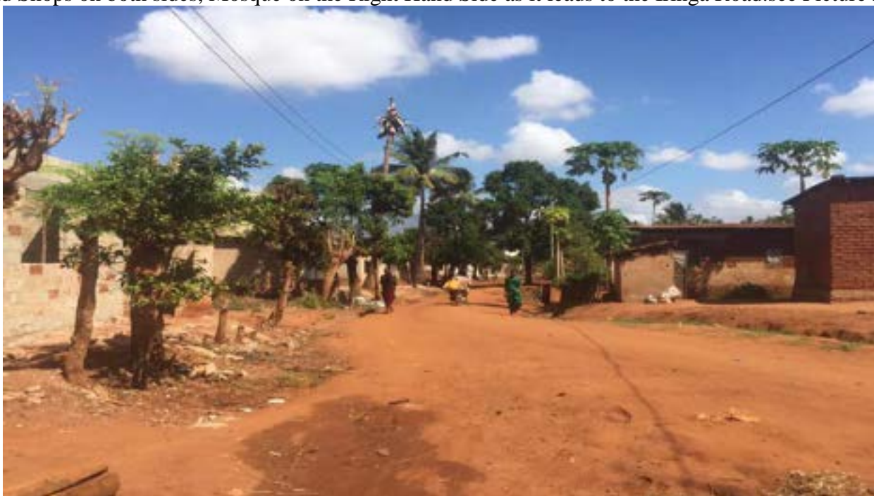
Picture 2-8: Condition of Existing Mapande Road
