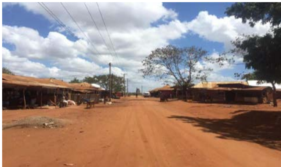
Picture 2-5: Condition of Existing Mjimwema Road Source: Site Pictures- December 2021
