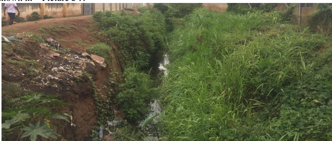
Picture 2-11: Solid Wastes and Vegetation along the Drainage Section
