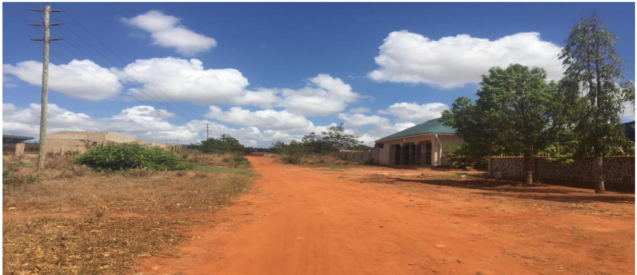
Figure 1.2:: Condition of Existing Muhimbili Road
