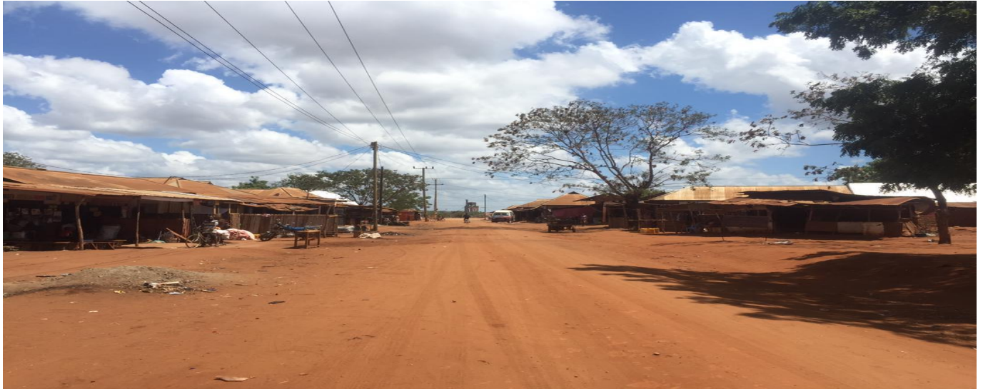
Figure 1.3:: Condition of Existing Mjimwema Road
