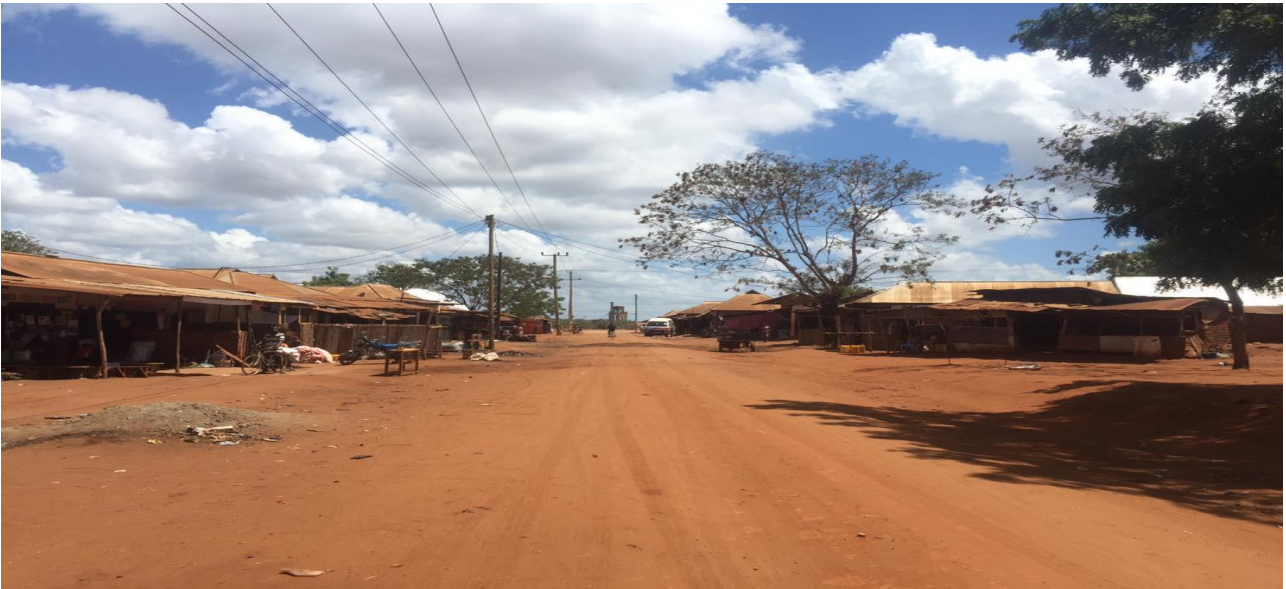
Figure 1.4: Condition of Existing Tubuyu II Road
