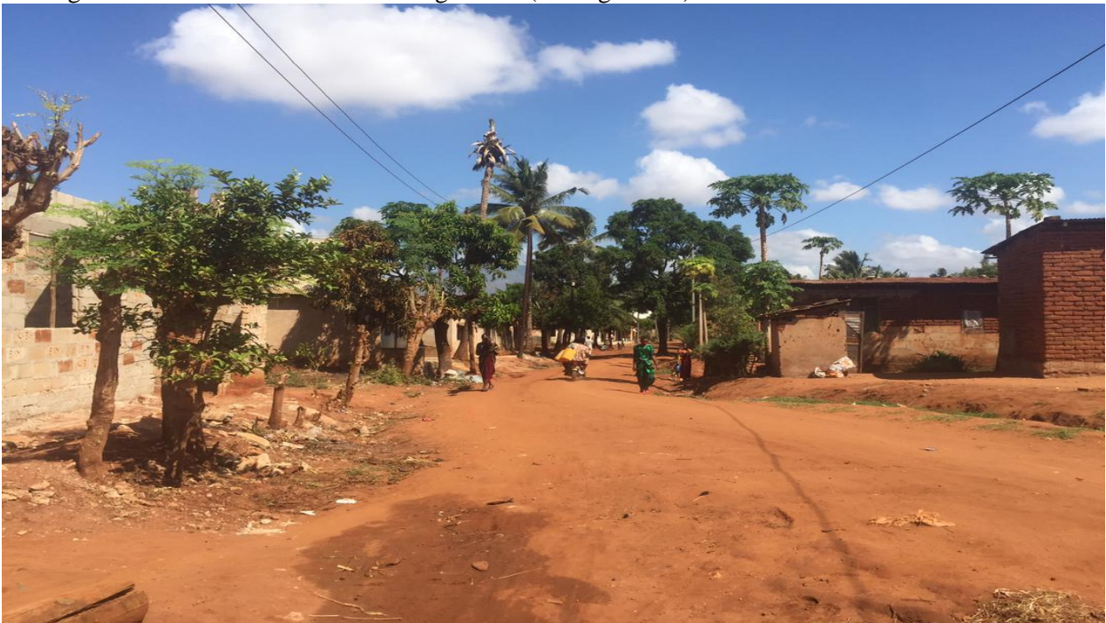
Figure 1.5: Condition of Existing Mapande Road
